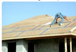
Secondary Water Resistant Roofing Installation
